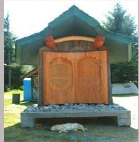
**A movable concrete pad with a Cedar Shake and timber roof is built to display each Log Book in the park.**
